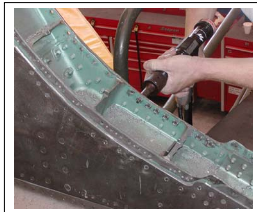
Figure 9: Use of ForceTec to Resize Ovalized Holes in a Leading Edge Spar
